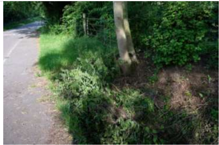
7.2 Blocked ditch opposite telephone exchange on Ingham Road
