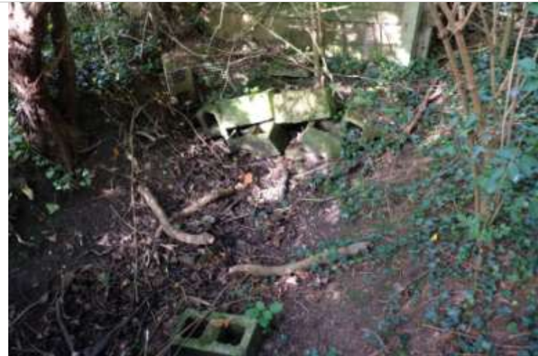
9.5 Clogged drain crossing footpath on north side of copse
